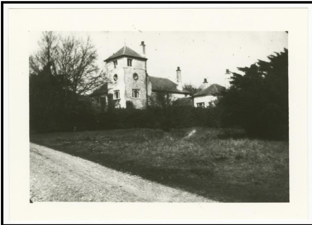
Beacon Hill: The tower.
